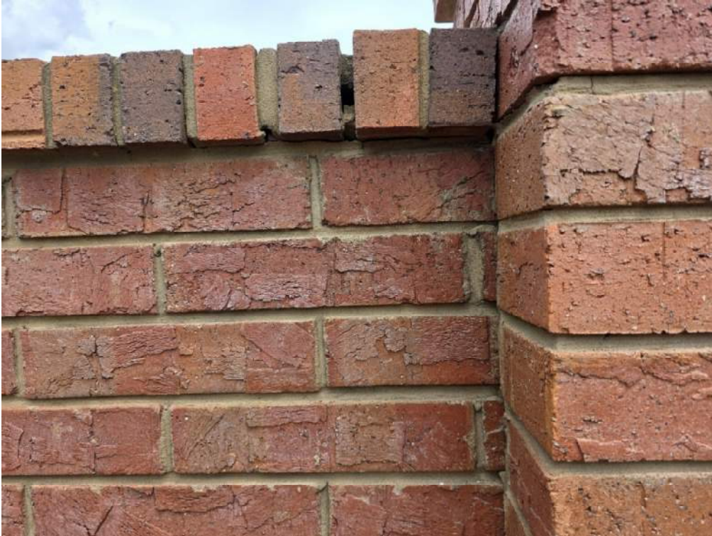
50 – Mortar cracking on cap
