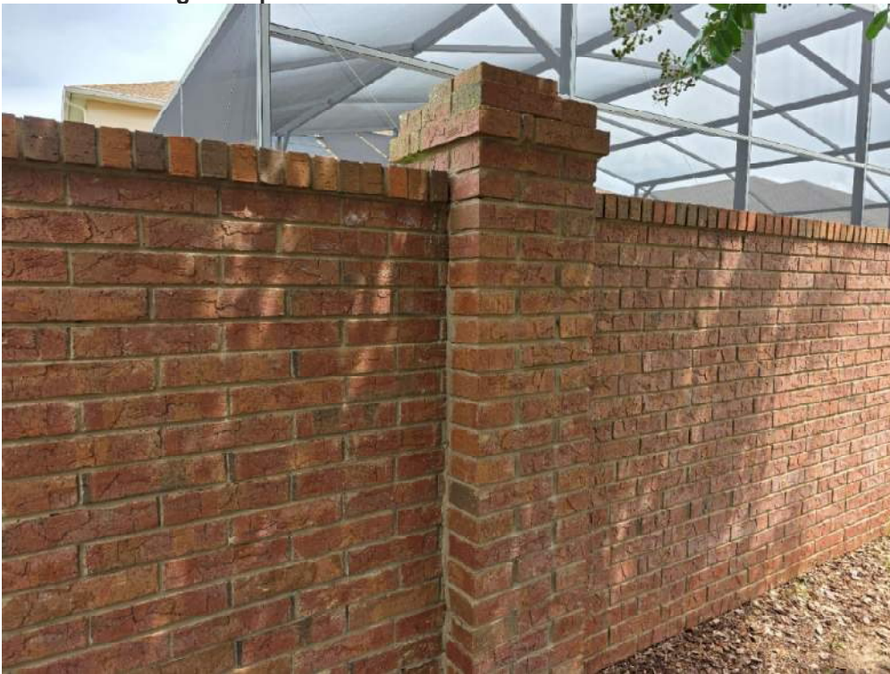
50 – Mortar cracking on cap
