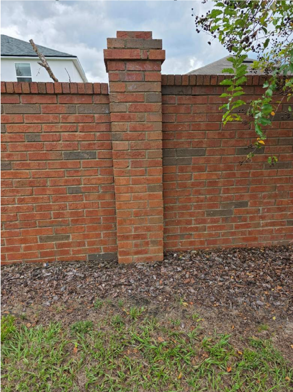
78 – Mortar missing between bricks; column damaged
