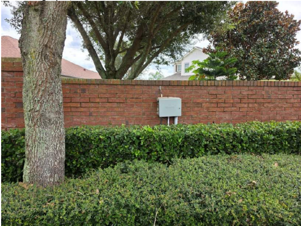
33 – Missing repair; irrigation box disconnected from wall.
