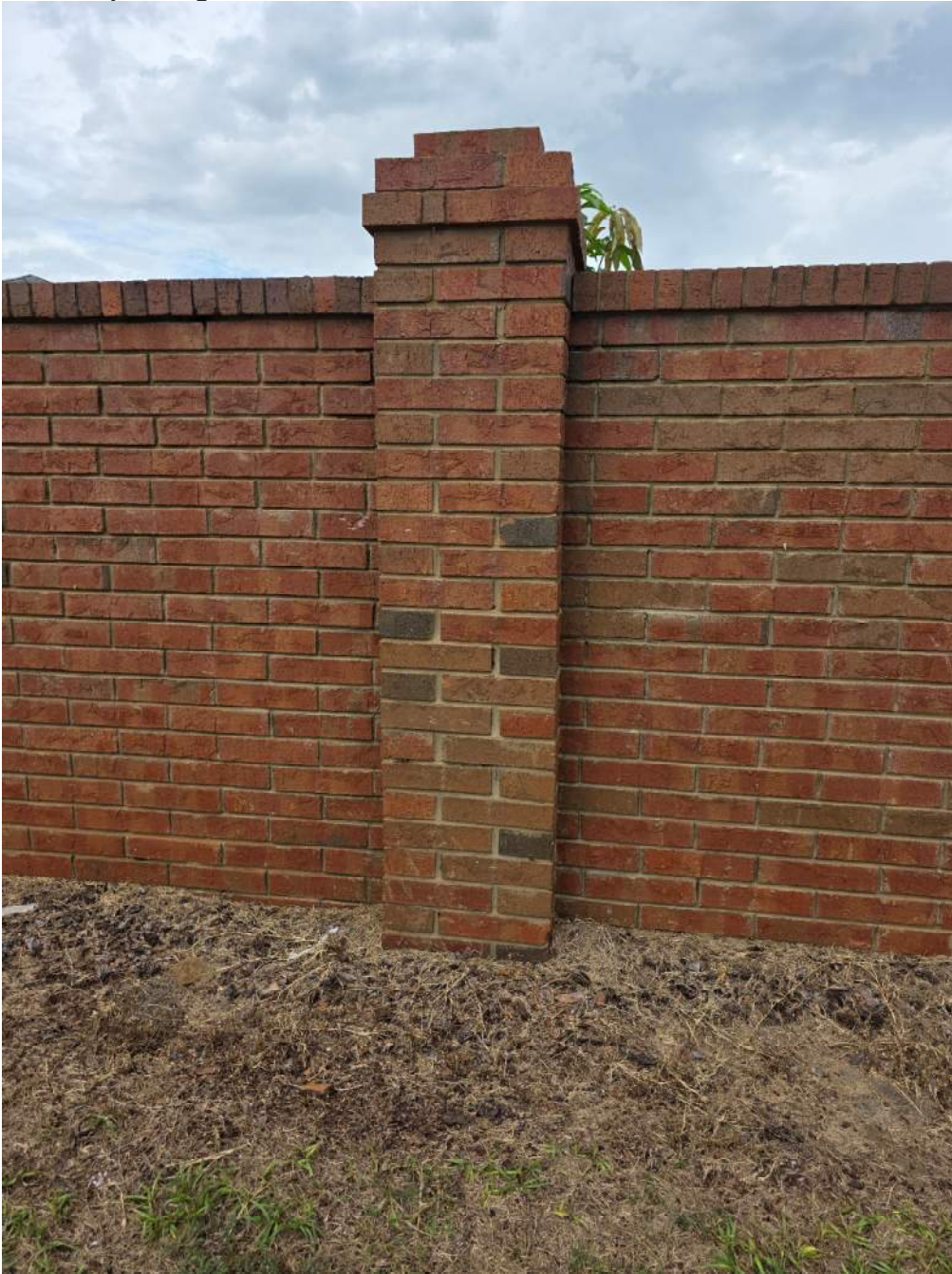
90 - Grout separating
